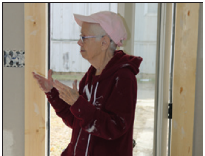
Sister Vickie Perkins surveys progress on the rehab of a DLAH house.
